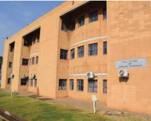
Sasol Computer Building
