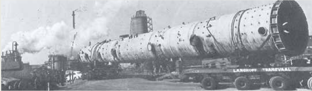
Rectisol Tower for Sasol
