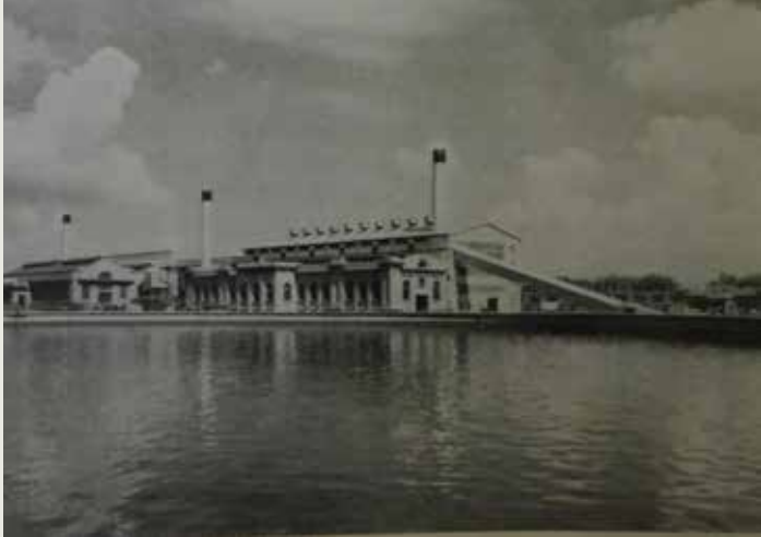
The pumping station at Vereeniging
